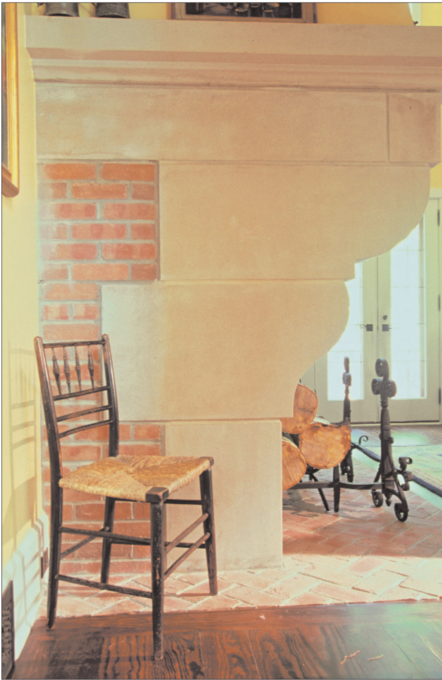
This chair in the living room reveals the scale of the corbelled limestone fireplace, which has a 60-in.-tall opening.
