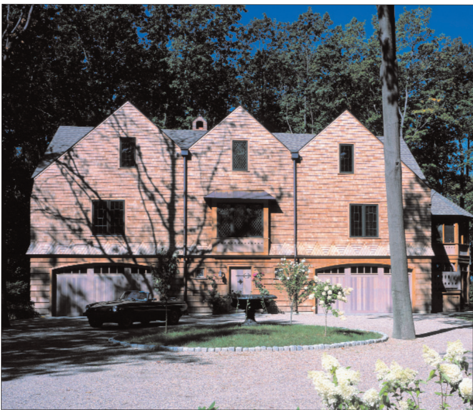
The main entrance to the triple-gabled Hayes cottage, in South Haven, MI, is quite formal, with the house sitting on the entry court. The exterior doors and garage doors were custom made in mahogany by Bruce and Paul LaRose, who did all of the millwork for the cottage, including the stairs, columns and the bed for the master bedroom.
