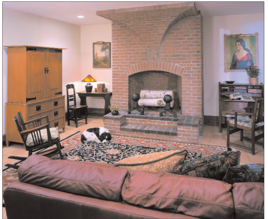
Constructed of salvaged brick, the vaulted fireplace in the ground-floor family room incorporates a hearth and a 12-in. original Batchelder tile at the vault's springpoint. The Ambrose Heal linen press on the left has been converted into a media center. Other furnishings include an antique Mission rocker and a slant-top desk by Limbert of New York City.
